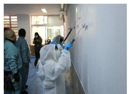
(校舎内壁塗り)
